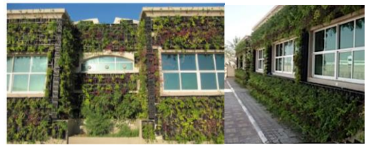
Figure 17, The irrigation system delivers Greywater to vegetation that drapes Liwa's external facades.
