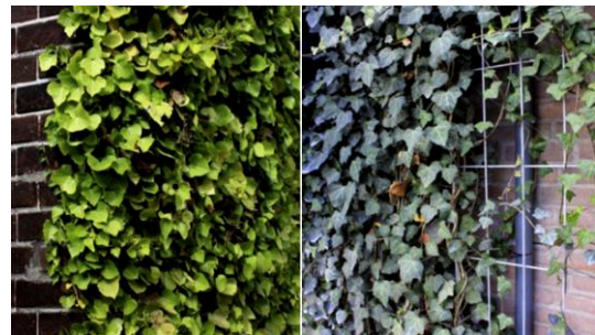
Figure 4, a. Direct facades (left), b. Indirect facades (right), (Source: [9])
