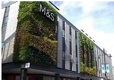
Figure 2, LWS, M & S Newcastle, UK (source: https://livingwalls.ie/gallery/ms-newcastle/ )
