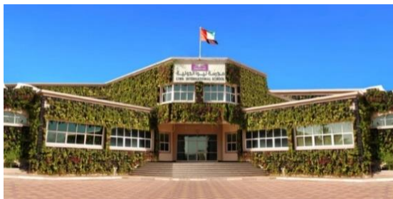
Figure 16, LWS, Liwa International School, Al-Ain, (Source: https://whichschooladvisor.com/uae/school-review/liwa-international-school )
