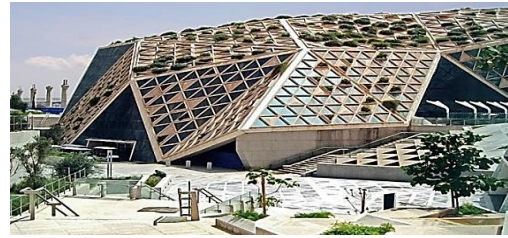
Figure 19: Exterior of KAFD (source: https://saudiprojects.net/wp-content/uploads/2018/04/conference_002.jpg )
